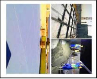
5. Screed in Panels & Slope
