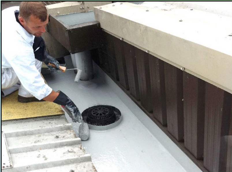
Roof Gutter GRP Lining
